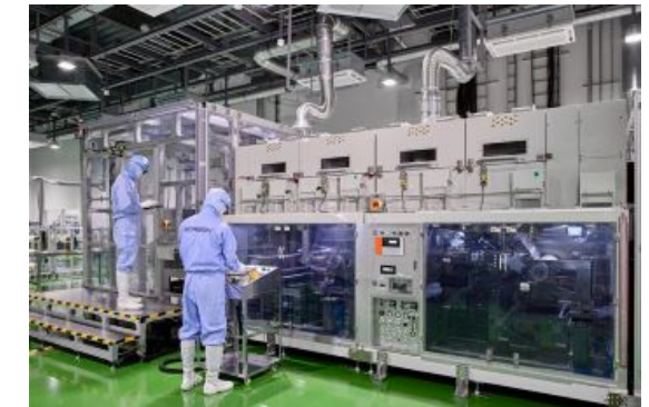
Mass-Production Facility for PEXEM™
